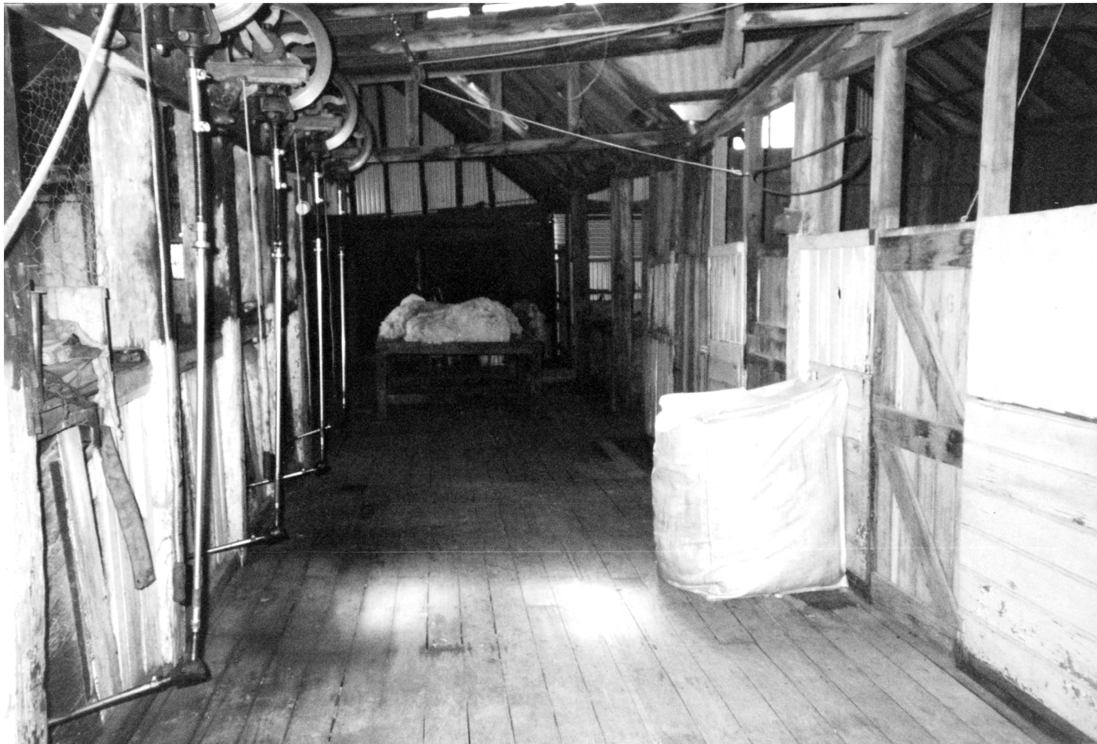
A photograph of the board of the woolshed viewed from the east taken about half way along its total length.
