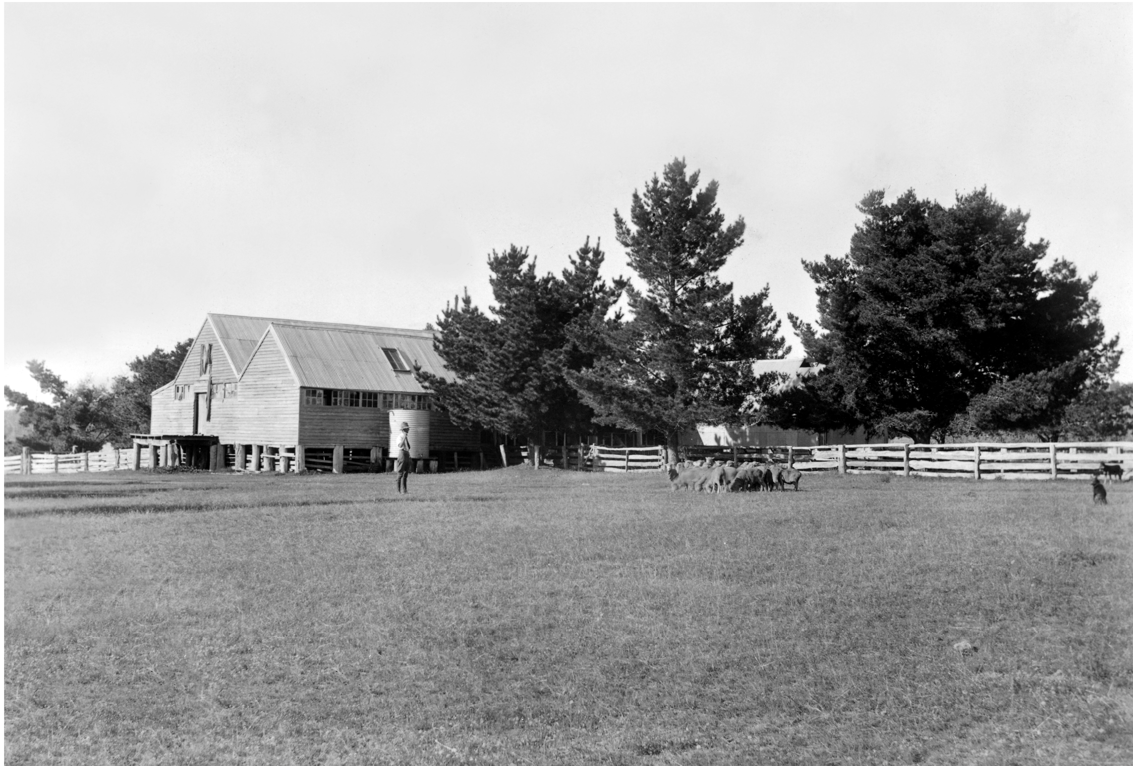
The Invergowrie woolshed viewed from the south-west, 1917.
